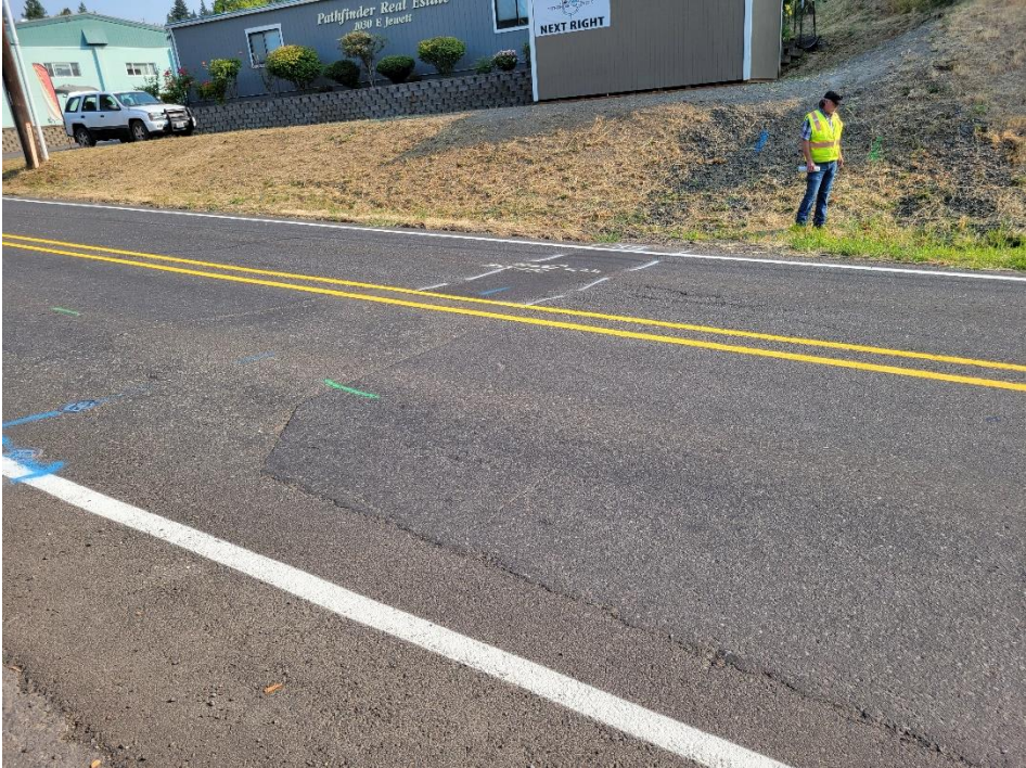
Photograph 8: E. Jewett – East of Ingram Place Tie-in Connection
