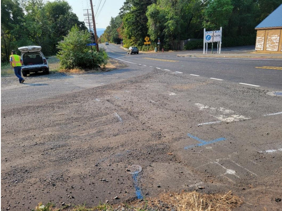
Photograph 5: Vine Street Crossing at East Jewett
