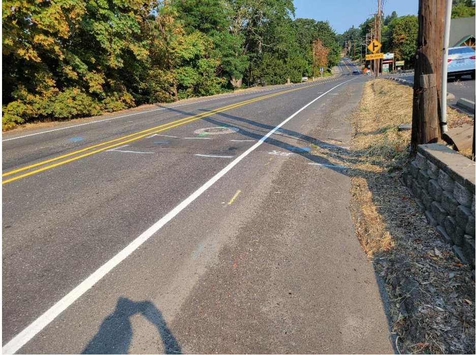
Photograph 7: 1000 E. Jewett Service Line
