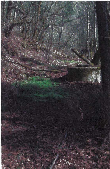
Concrete Diversion Vault
