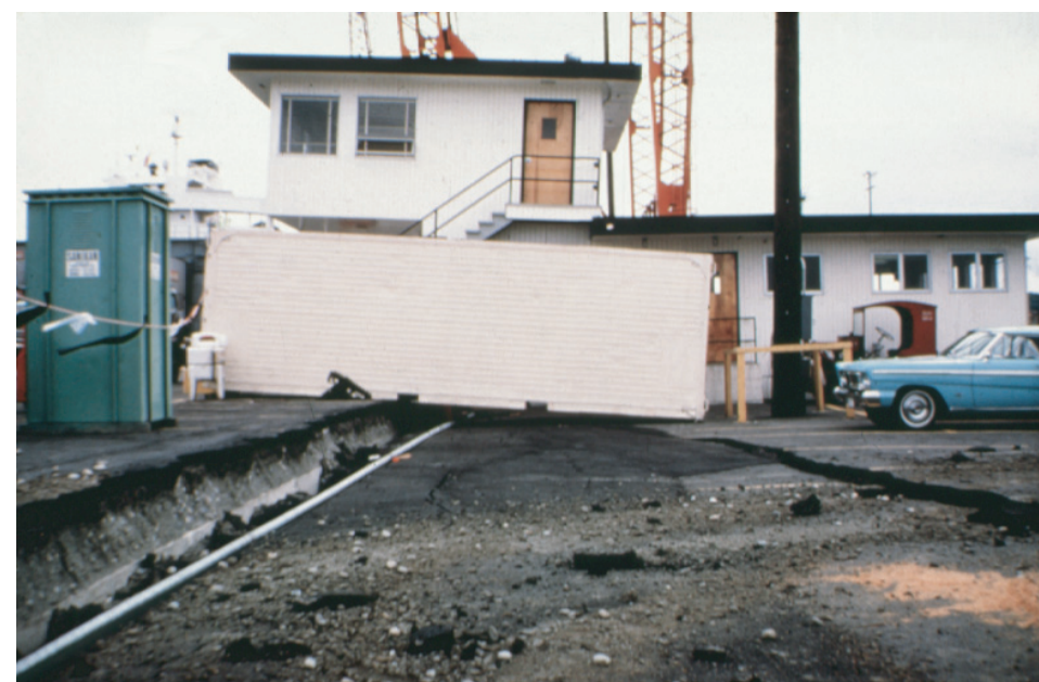
Liquefaction during the 1965 Seattle earthquake caused both lateral and vertical movement of the ground in the Port of Seattle. Cargo cranes such as the one in the background are vulnerable to liquefaction-induced ground displacement. Lateral spreading such as this can cause severe damage to both above-ground structures and underground utilities. Photo courtesy of the Karl V. Steinbrugge Collection, Earthquake Engineering Research Center [http://nisee.berkeley.edu/visual_resources/steinbrugge_collection.html].
