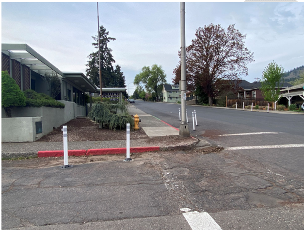
Some streets that do have sidewalks do not have curb ramps at corners, even where marked crosswalks are striped. Maintenance of existing roadways remains a priority for the City.
