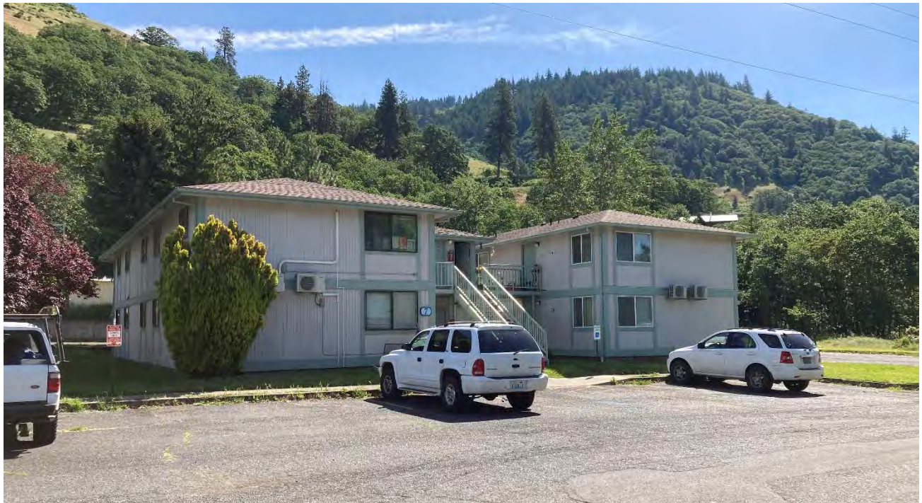
Photo 2. View northeast showing parking area and typical 2-story residential building.
