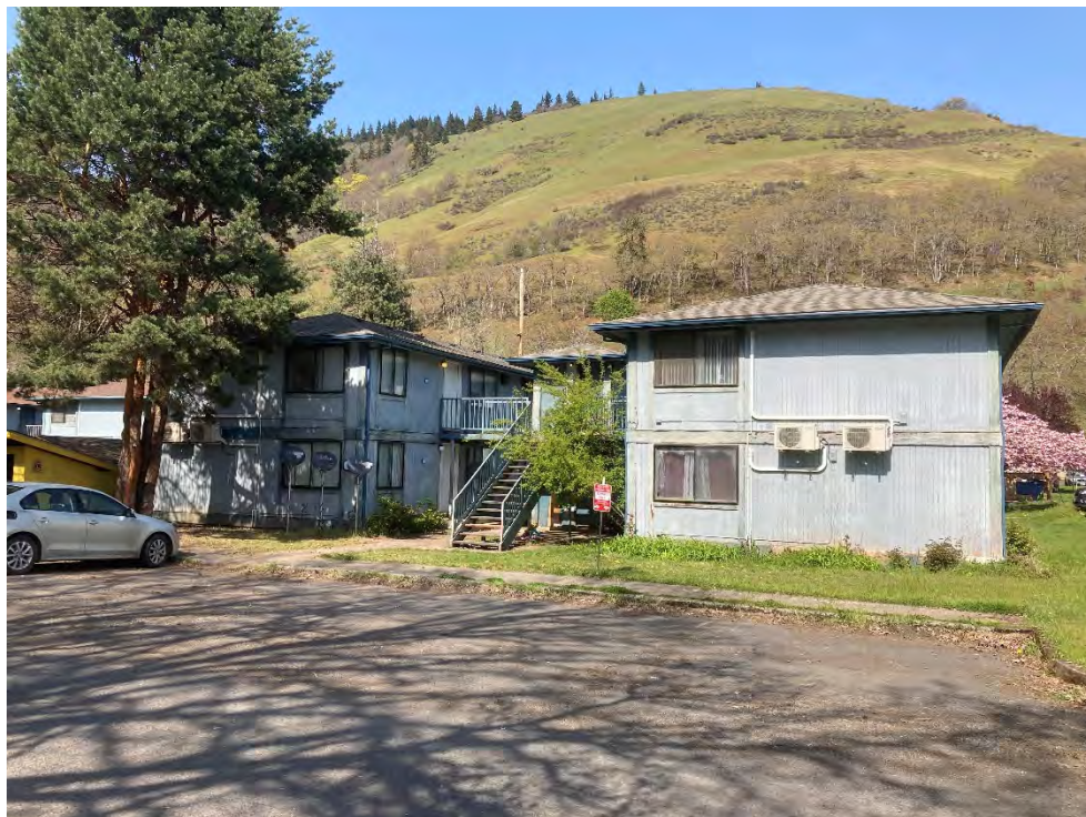
Photo 2. View toward the north showing stairs to second floor apartments.
