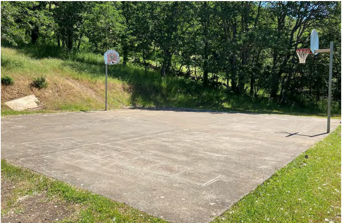
Photo 6. View northeast of basketball hoops at the NE end of the project area.
