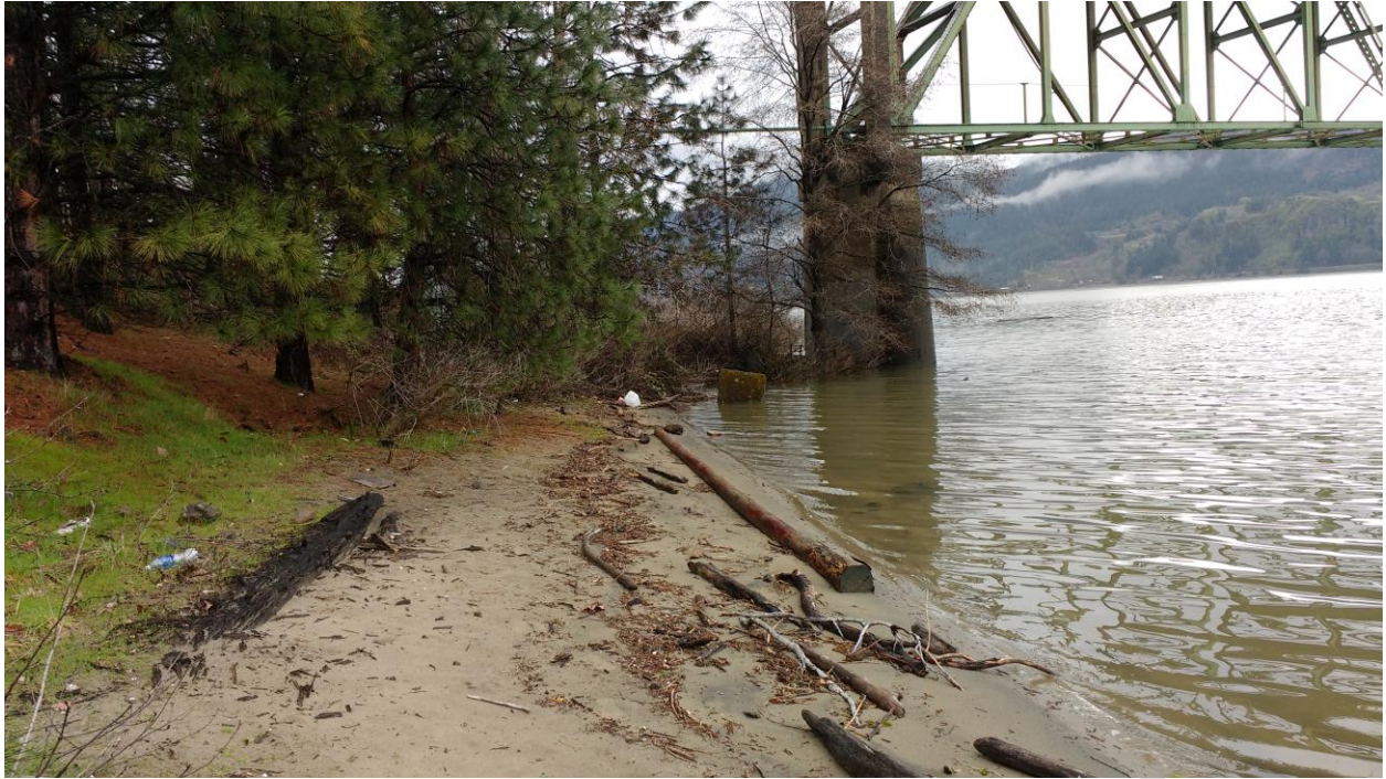
Beach downstream of Hood River Toll Bridge
