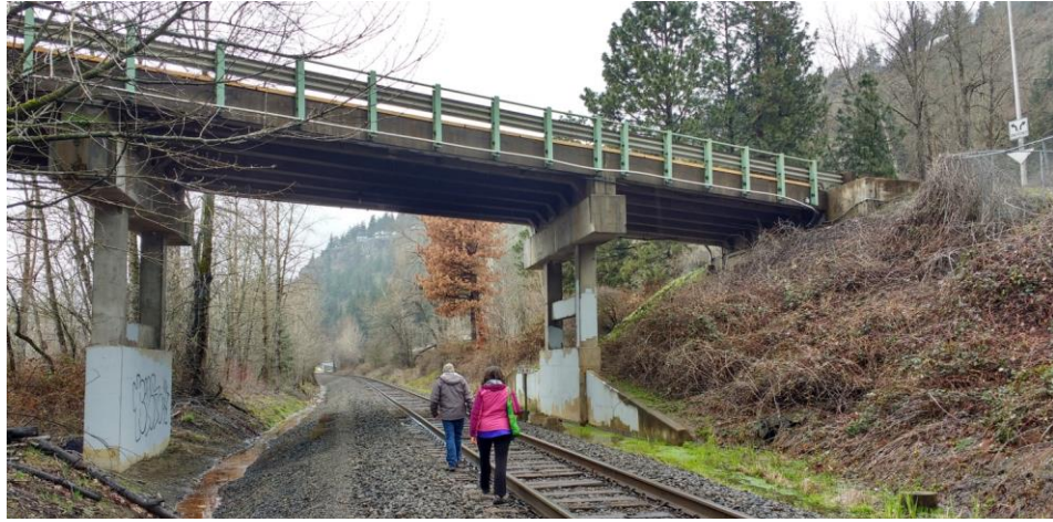
BNSF Railroad & Hood River Toll Bridge
