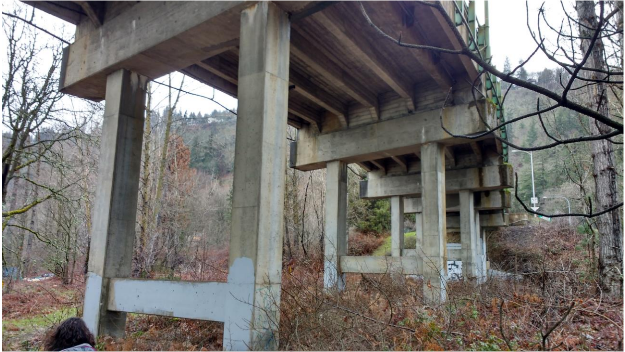
Underneath Hood River Toll Bridge
