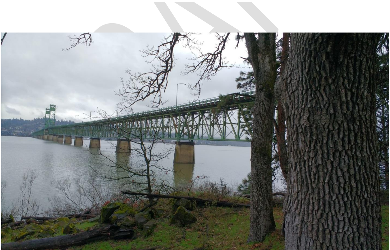
Looking at Hood River Toll Bridge from the northeast
