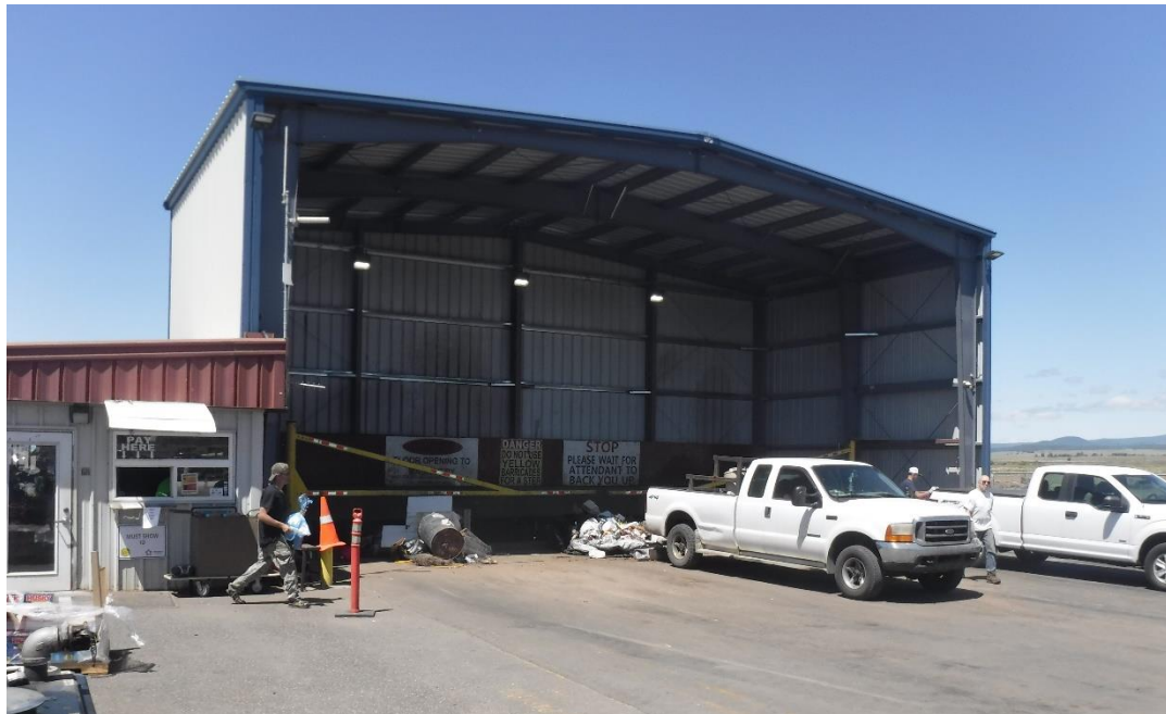
Figure 6-3. Goldendale Transfer Station
