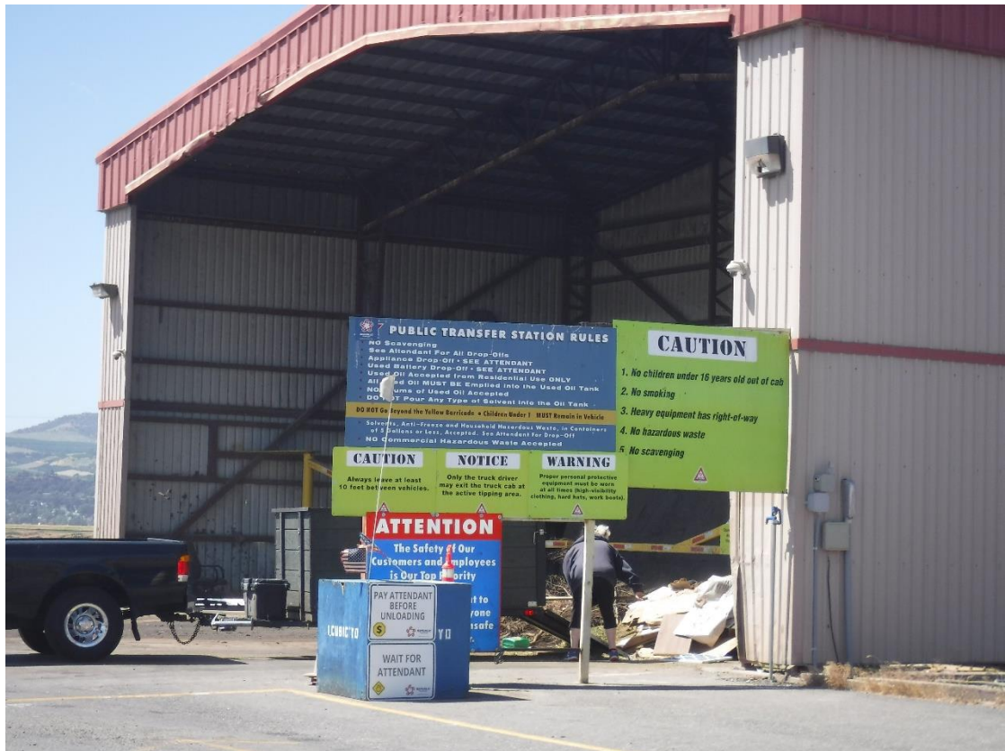
Figure 6-2. Dallesport Transfer Station
