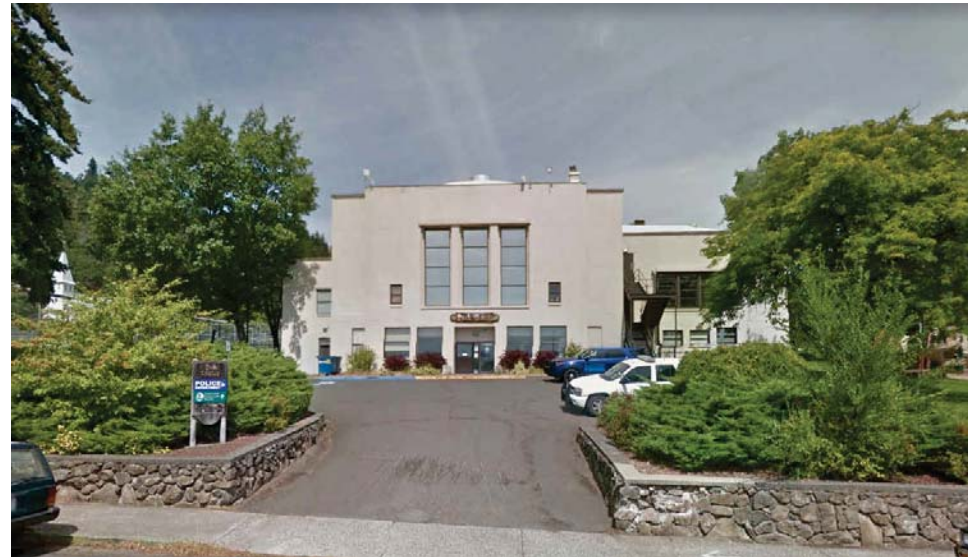
"PARKS" BUILDING, SOUTH ELEVATION VIEW
