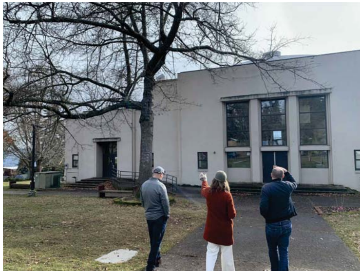
"PARKS" BUILDING, NORTH ELEVATION VIEW
