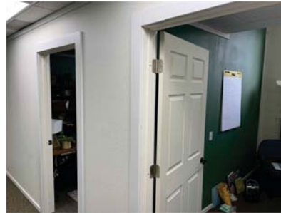
1 - DOORS AND WALLS WITHIN THIS IMAGE ARE TO BE DEMOLISHED
