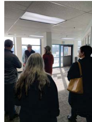
4 - LOWER LEVEL ENTRY - WALL TO RIGHT TO BE DEMOLISHED
