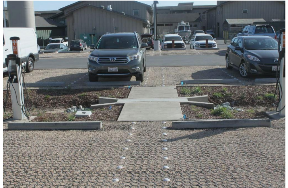
Plastic Grid pavers hold gravel in place
