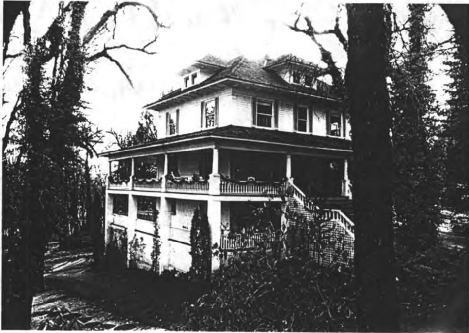
Figure 19. HSN-5, Building 1, looking to the southwest.
