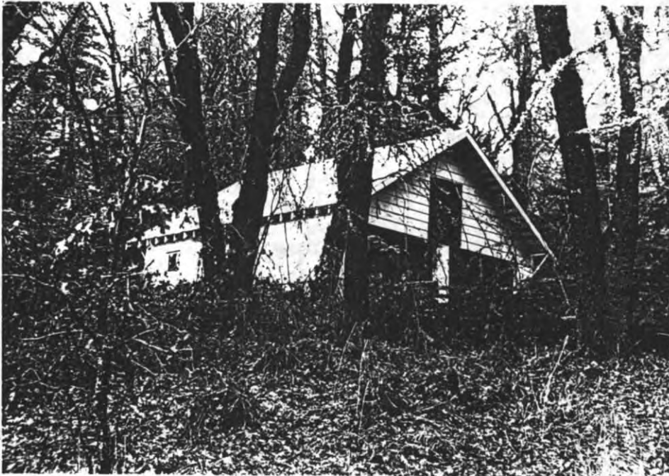
Figure 20. HSN-5, Building 2, looking to the northwest.
