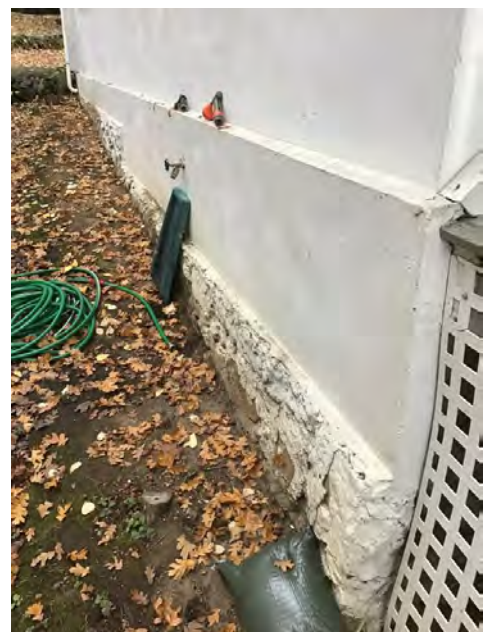
West side foundation area-
