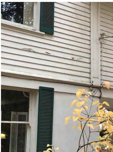
West Side SW bedroom wall
