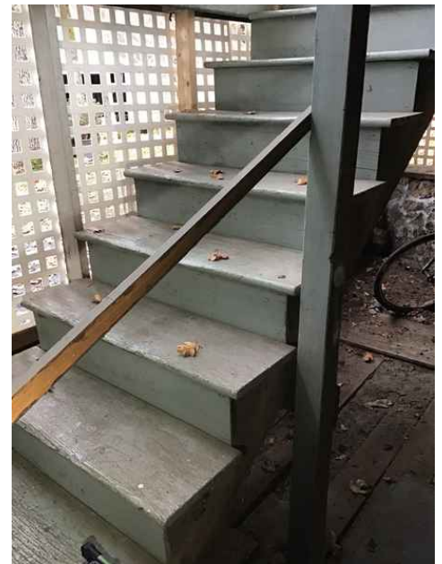
Rear lower S Side stairs
