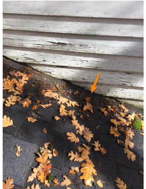
South bath dormer roof contact
