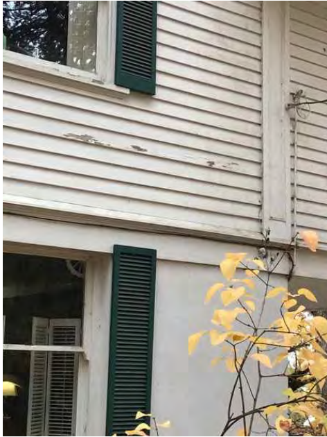
West Side SW bedroom wall
