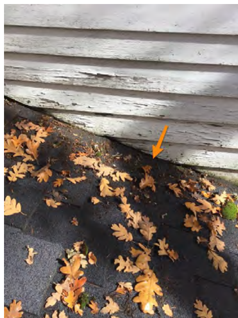
South bath dormer roof contact
