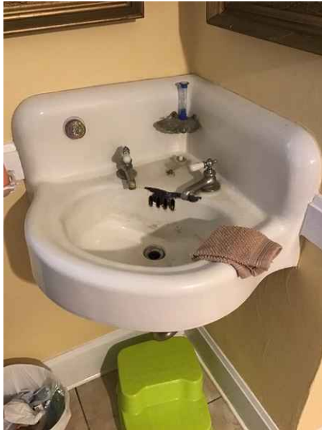
Older corner sink with damage (chipped) noted. No shut off valves noted below the sink.
