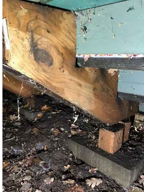
At the lower areas of the N steps
