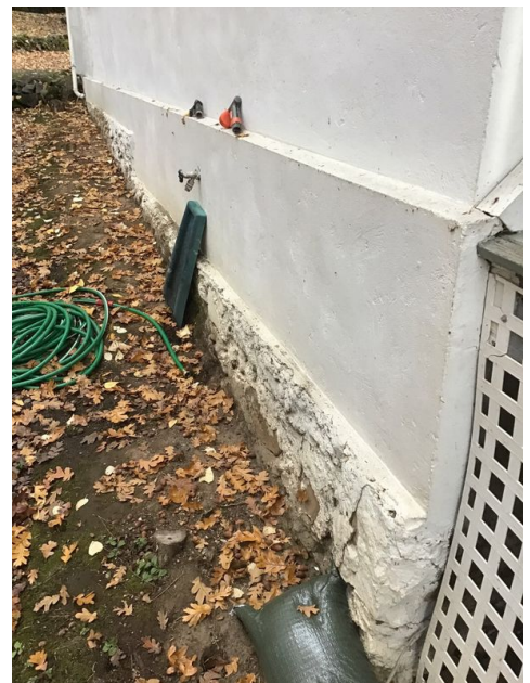
West side foundation area-
