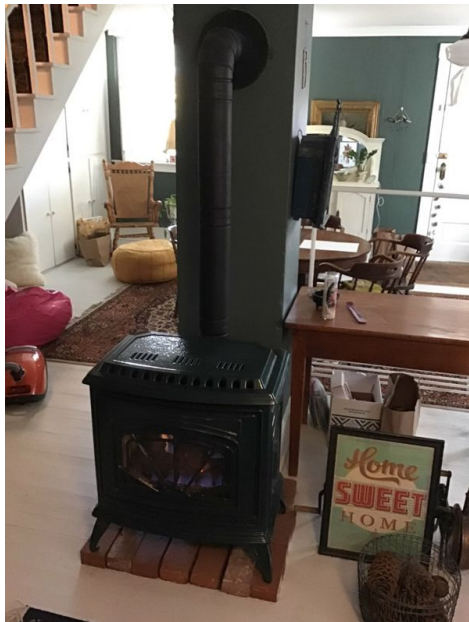
Lower level unit - Appears to function
