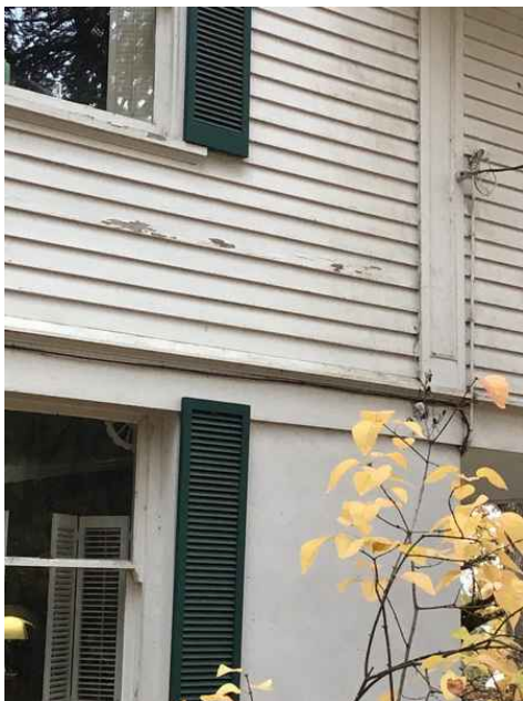
West Side SW bedroom wall
