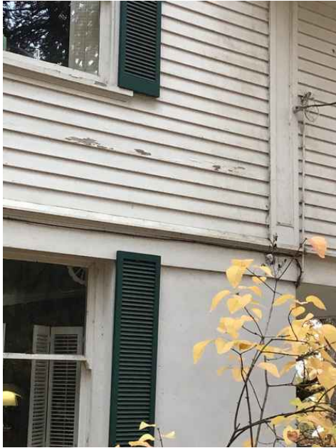
West Side SW bedroom wall
