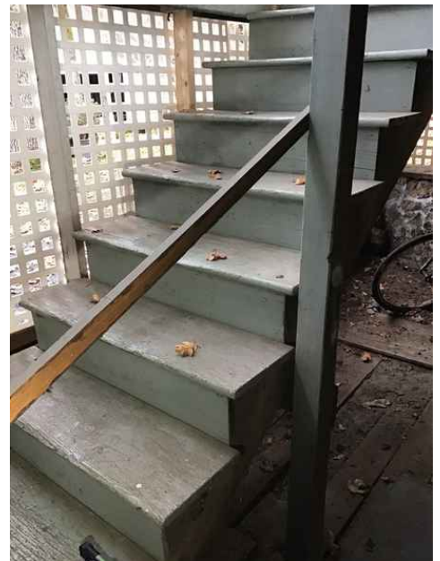
Rear lower S Side stairs
