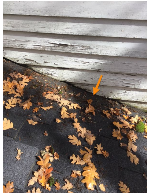
South bath dormer roof contact
