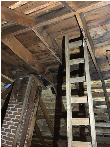
Indications of past leaking noted- None at the time of the inspection.
