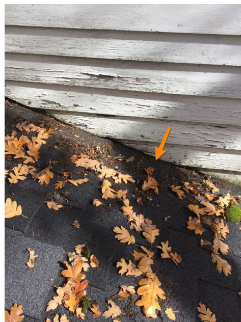
South bath dormer roof contact
