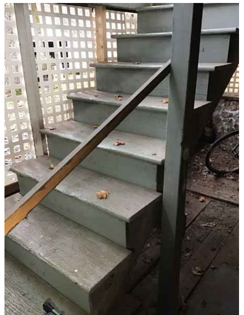
Rear lower S Side stairs
