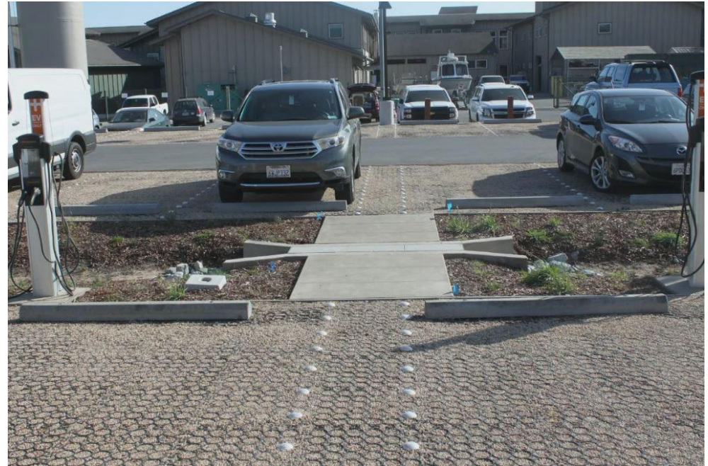
Plastic Grid pavers hold gravel in place
