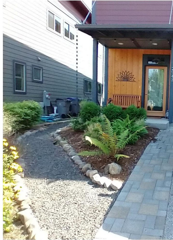
Hood River rain chain and pervious paving
