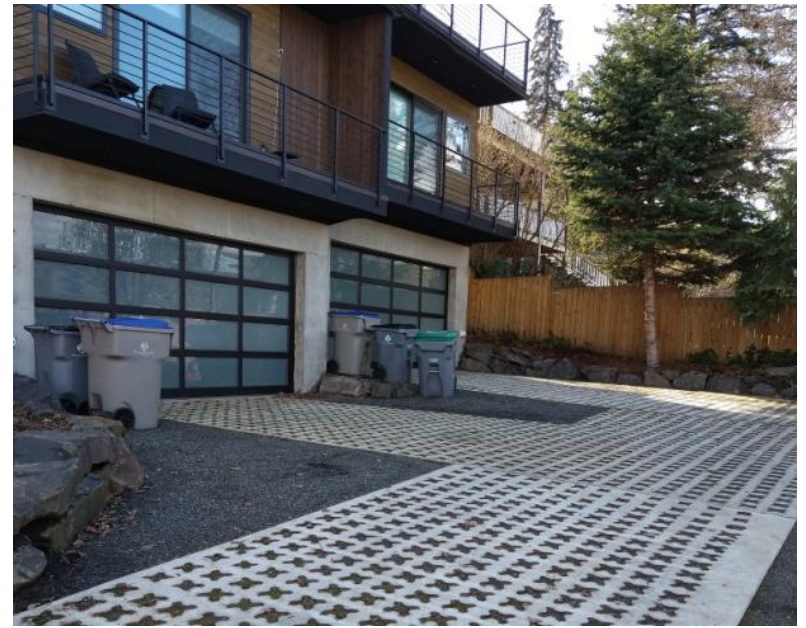
Code approved driveways Hood River
