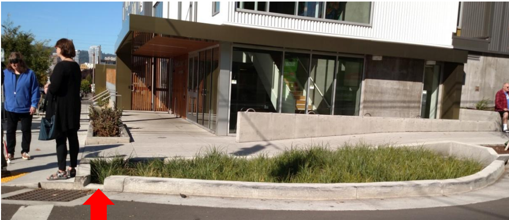
Curb cut to planter Portland OR
